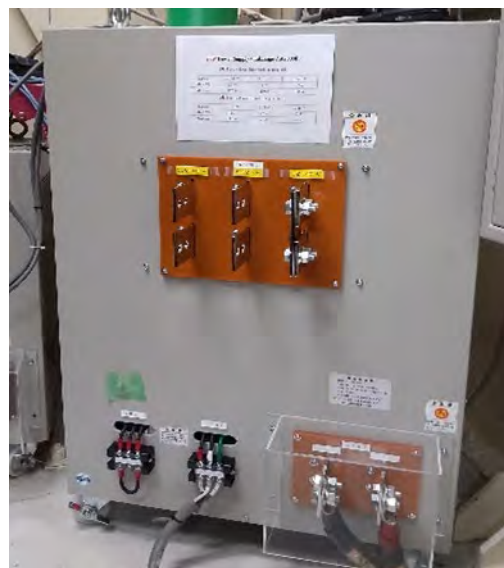
Fig. 3. Newly installed transformer at optical hutch 3, BL04B1.
